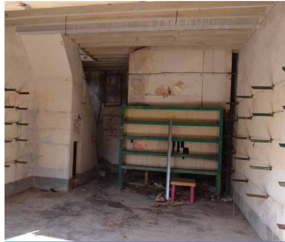
木地板欄柵 Timber floor joists
