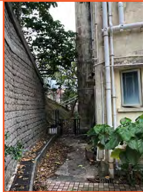
護土牆 Retaining wall
