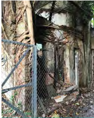
磚牆 Brick walls
